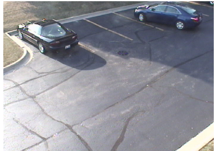
Great Color Video and High Speed Camera Control for Home or Business Security Camera Installations
